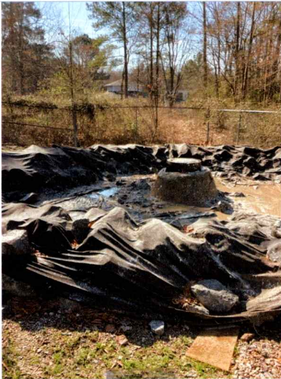
MH 1866 After Cleanup
