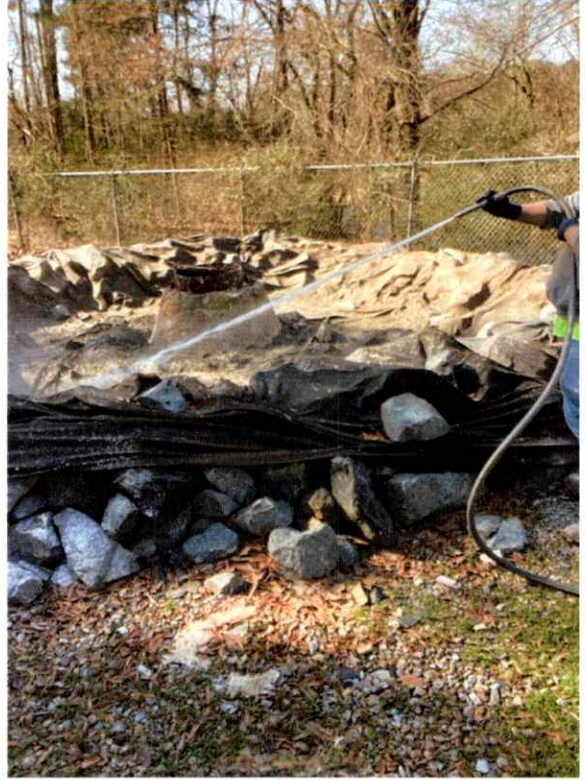
MH 1866 During Cleanup -
